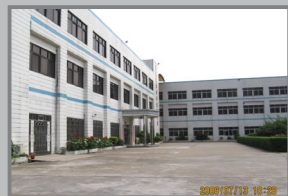
2008 Building of 25000m3 new plate in Fangqiao.
