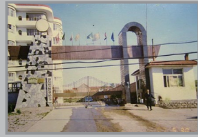
1998 Establishment of Josense refrigeration Equipment Co., Ltd by Mrs Li
